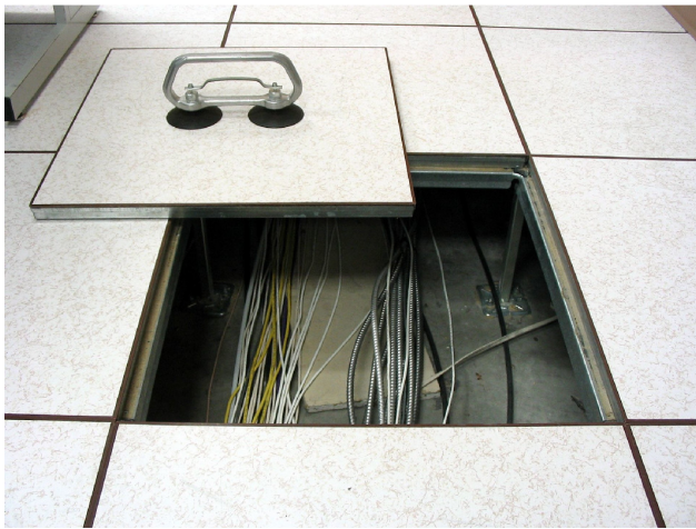
Figure 2.3: A raised floor creates a hidden void for the passage of cables.
